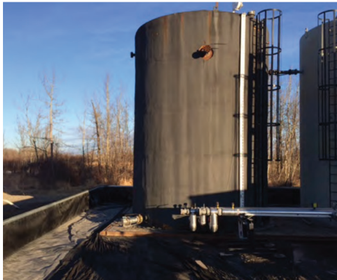
Figure 3. Lined steel dike (secondary containment)
